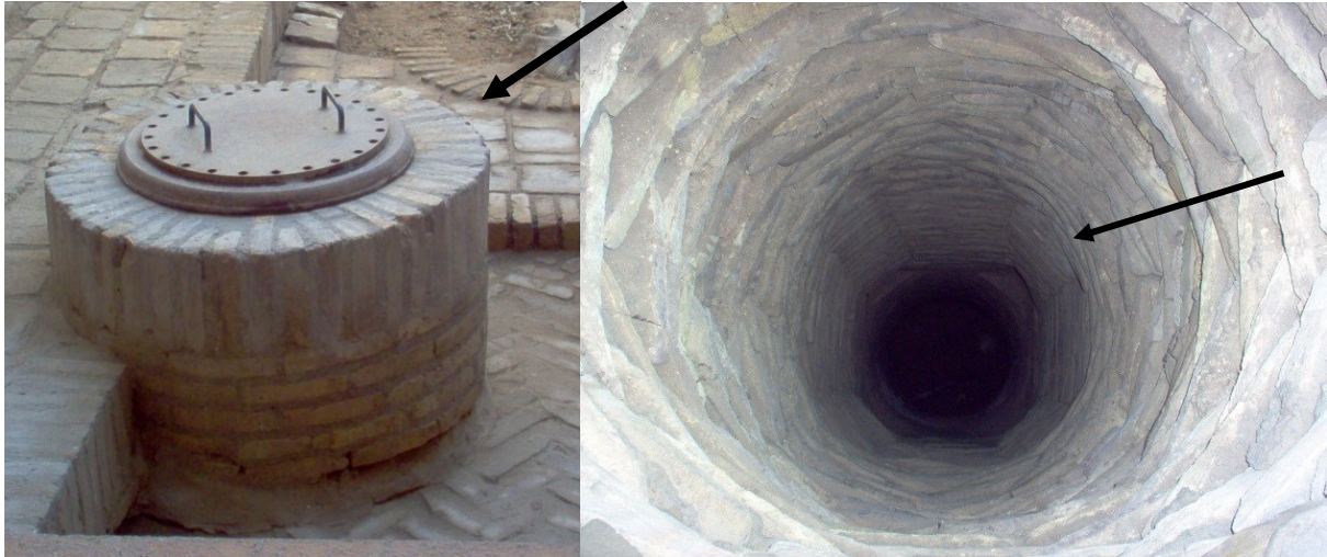
Figure 7. These are the current views of the well. The top part of the well was later rebuilt with burnt bricks and the inner part was remained as it was before. Photos taken by author.
