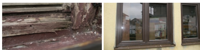
Figure 2.9. Old (left) and new windows (right)
